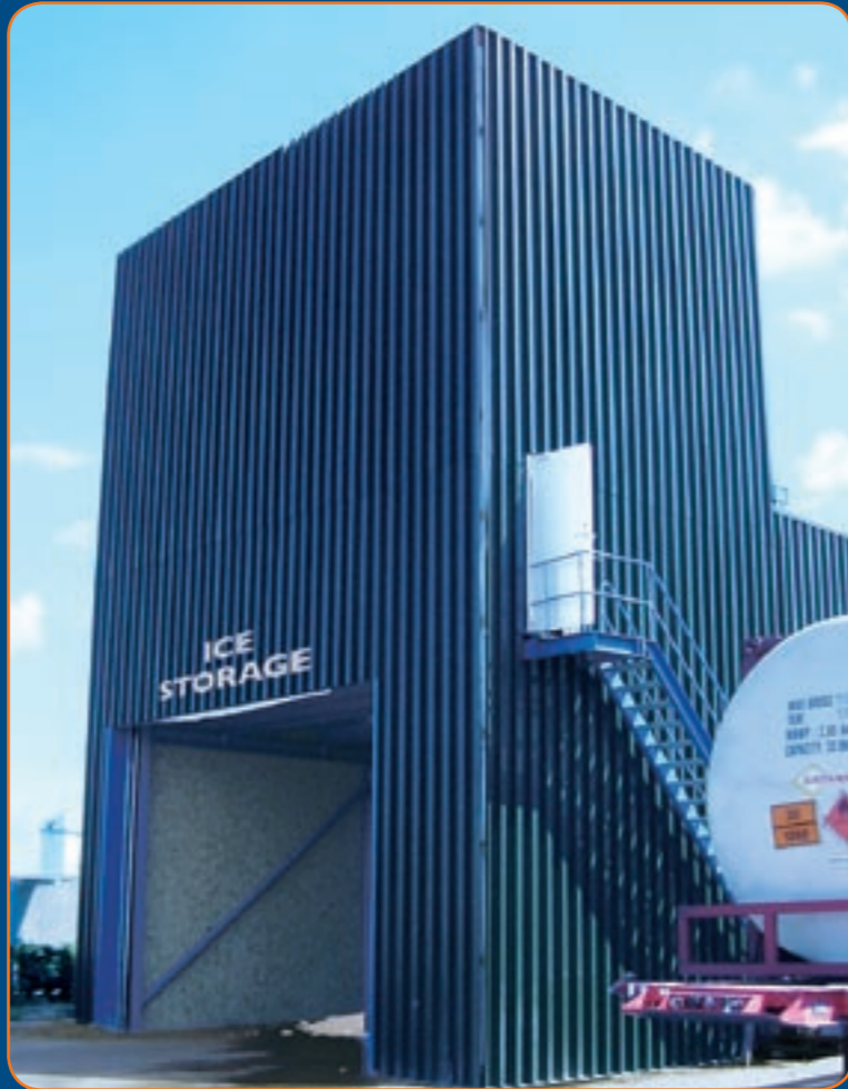
Ice Storage for delivery of ice to trucks or into bins. A conveyor for delivery of ice into icedoser can also be delivered as optional equipment
