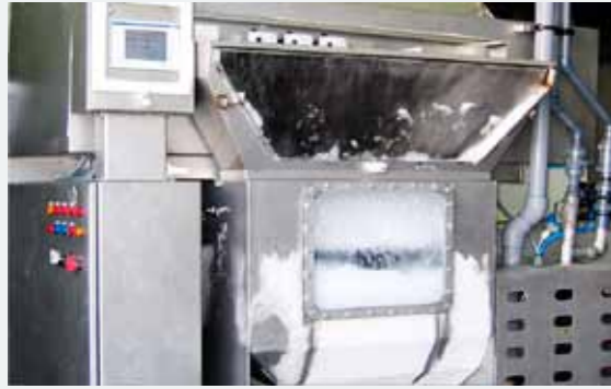
1.1 - Fluid Ice system: Ensures maximal cooling and increases capacity of Super Chiller.
